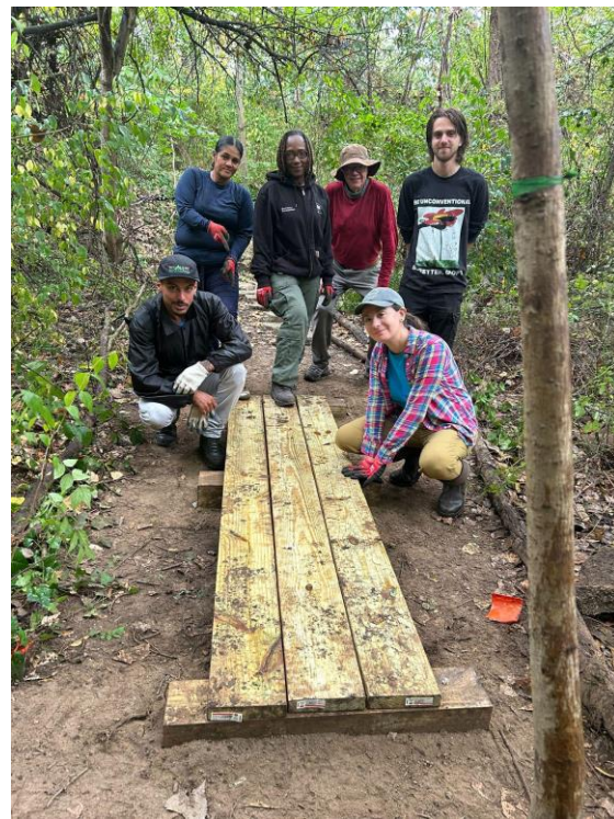
Figures 1 & 2. NAC staff and partners showing turnpike they installed as part of 2024 trails techniques training; NAC staff and partners showing puncheon they installed as part of 2025 trails techniques training.
