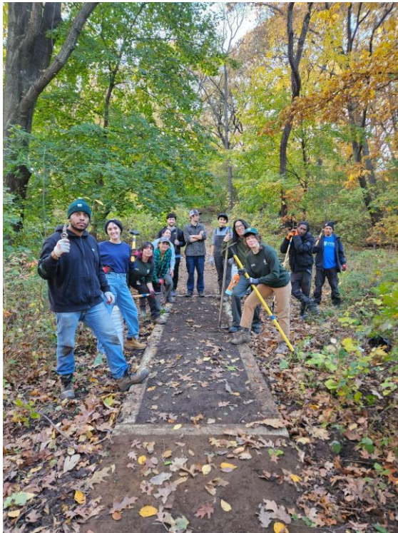
Figures 1 & 2. NAC staff and partners showing turnpike they installed as part of 2024 trails techniques training; NAC staff and partners showing puncheon they installed as part of 2025 trails techniques training.
