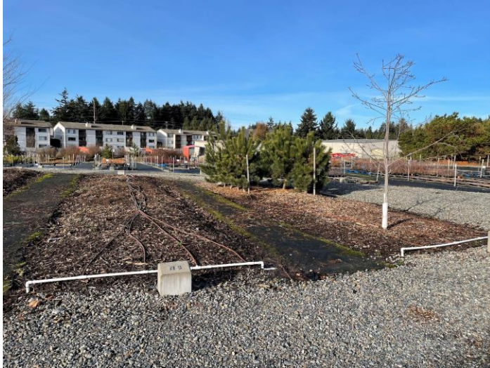
Figures 10–12. Row conversion in progress and after initial earth moving and gravel filling. Example of in-ground row setup prior to conversion.
