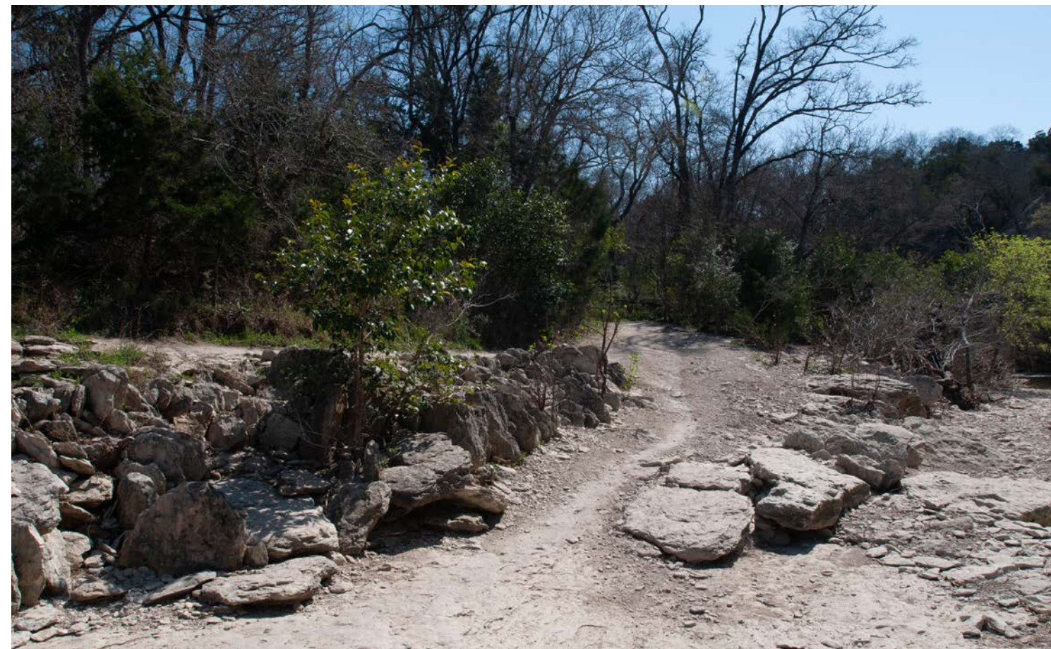
An armored bank at a water access point
