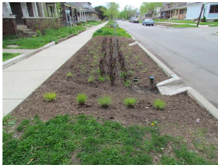
Rain garden, or bioretention basin, at Jefferson Avenue on the Near East Side
