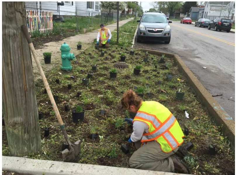
A rain garden, or bioretention basin, at Lincoln St. and Alabama St. on Indianapolis' south side
