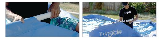
4. Insert the Pins down through the top of the T-Fittings until the Pins snap into place on the lower side of the T-Fitting.
