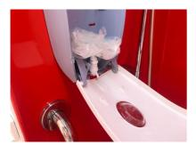
Remove the section of packaging as shown and align nozzle as shown.
