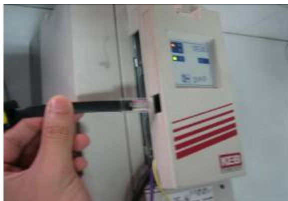
Fig2.2.3(2) Connect the DK1 module with an end of HSP5 line
